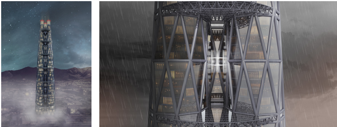
Figure 1: Render views of the proposed concept for a bundled tall building applied to a 320 m -tall case study in Pisa: overall view and detail of the vertical axis wind turbine.
